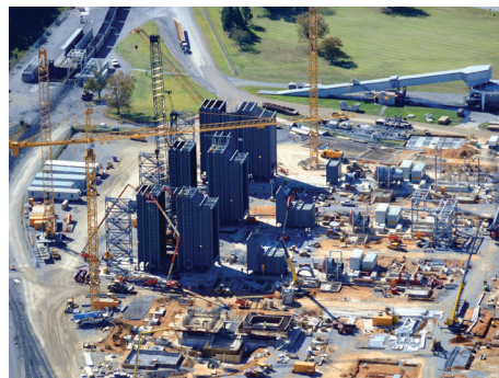
Casing being installed for all three units
