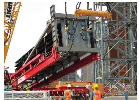
Two crane large module lift
